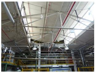
Figure A4.3: Interior of Factory #1 with butterfly roof
