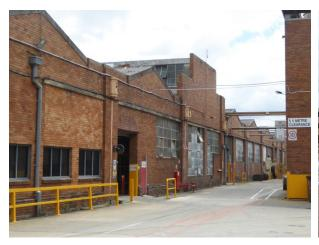
Figure A4.1: External view of the eastern side of Factory #1. The original c.1941 elevation was demolished and the factory extended east by 1961
