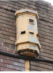
**Figure A4.6:** Detail view of a galvanised iron rainwater hood
