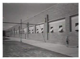
**Figure 1.9**1945 photograph showing the original factory building, west elevation. Note the incorporation of the rainwater heads into the design of the engaged piers and the expressed concrete lintels *Source: SLNSW, April 1945 (d1-39793h)*
