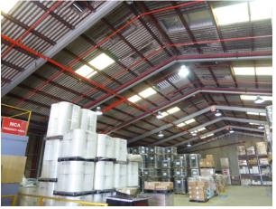
Figure A6.3: Interior view showcasing the steel portal frame structural system
