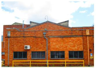
Figure 1.25 Image of the original Factory No.1, east elevation, showing the gable parapet and the 'butterfly' roof behind
