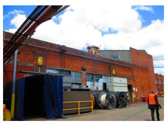
Figure 1.27 West elevation of Factory No.1 at the south end, showing the original engaged piers and rainwater goods, and the intrusive higher addition on the right with the metal wall cladding. The Administration Building is on the far right
