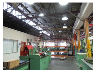
Figure A15.3: Interior of the north addition ahowing the saw tooth roof
