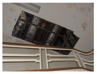
Figure A2.5: Section of ceiling in the first floor of the admin building removed due to water ingress damage
