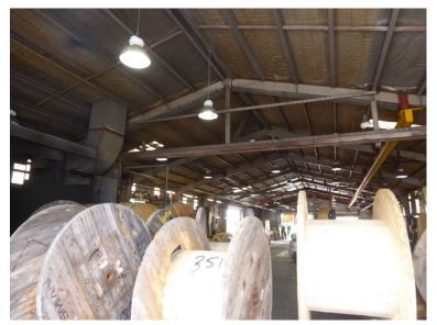
**Figure A25.1:**Portal frame interior of Cable Testing Building. Note the steel frame gantry structure in the foreground
