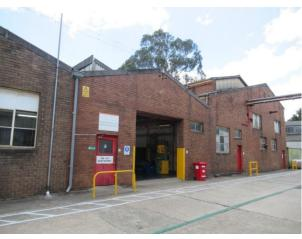
**Figure A15.2:** East façade of the Engineering Shop showing the later north addition to the building
