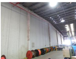
Figure A6.4: Later addition tilt up concrete panels seperating the original factory from the later addition
