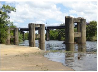
Figure 5.12 The concrete pylons to the former Liverpool footbridge and railway bridge
