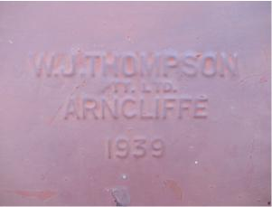
Figure A14.4: Embossed fabrication information on a fire door to the building
