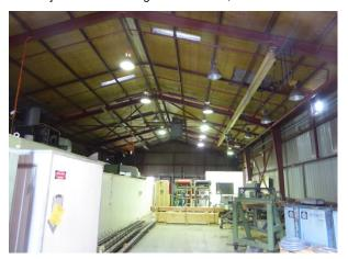
**Figure A8.3:** Steel portal frame structural system of Factory 5
