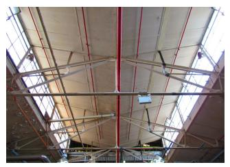
Figure 1.26 Image of the interior of Factory No.1, showing the 'butterfly' roof and clerestory windows
