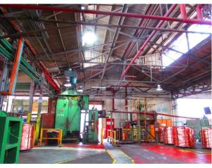
Figure A5.4: Interior of Factory 2 showing the structural system and butterfly roof
